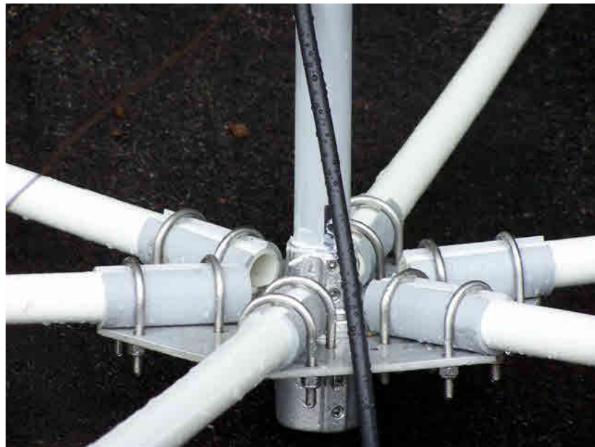
Close up of central hub that holds the spreaders. Very strong aluminum with stainless u-bolts
