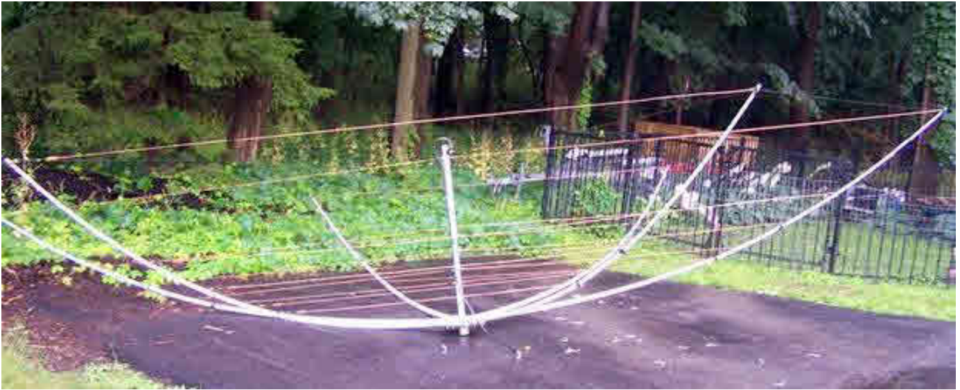
Antenna just after completion - on the ground Notice that the element wires are on the front and rear sides with just stabilizing Dacron lines from front to back
